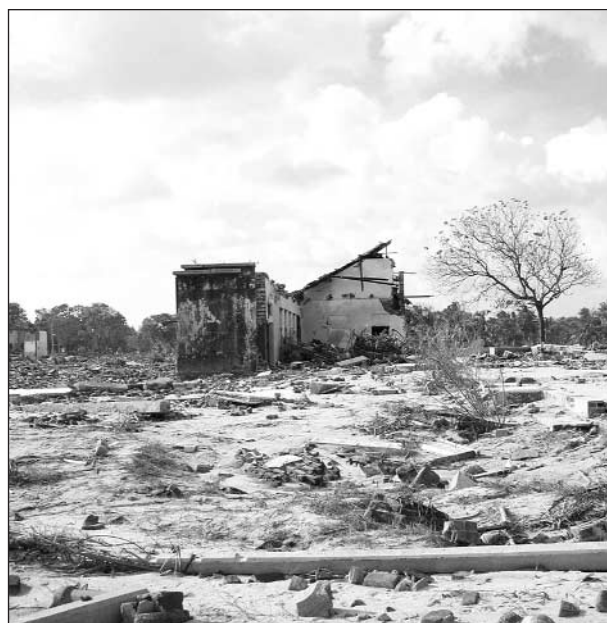
FIGURE 5 A damaged building near Kalmunai in Sri Lanka.
