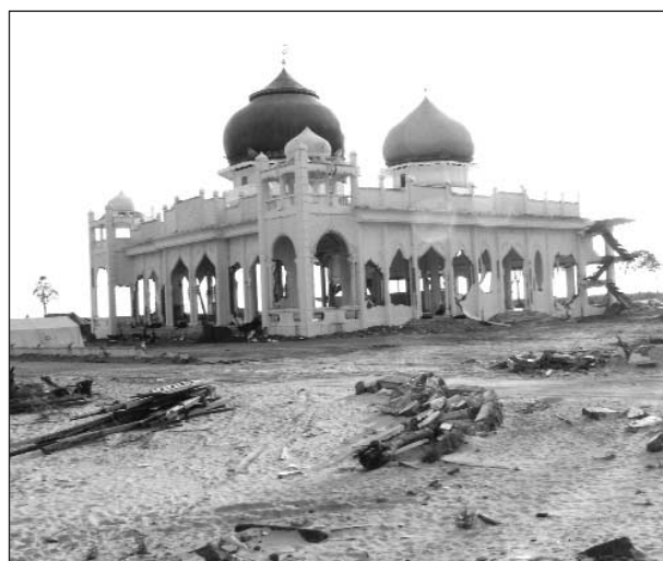
FIGURE 10 Photograph of a mosque in Banda Aceh showing that well engineered buildings survived the devastation.
