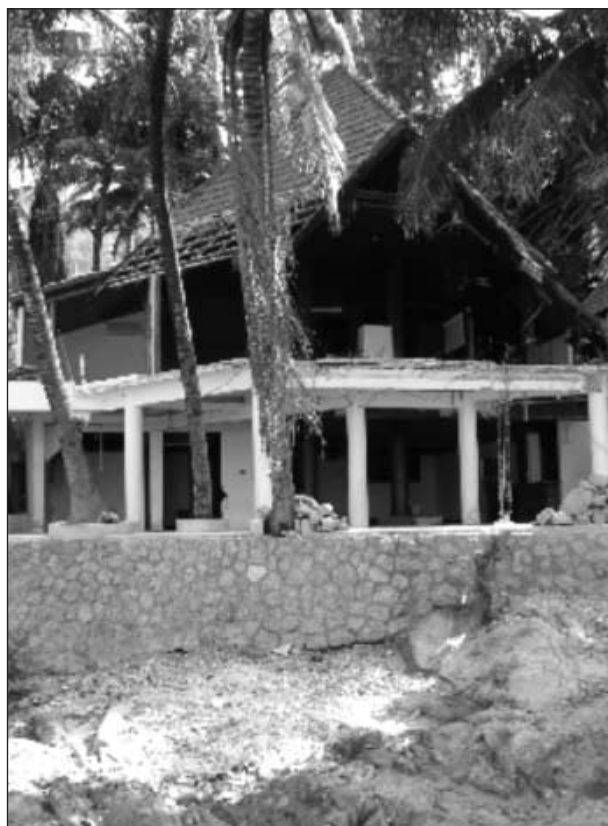
FIGURE 8 This seawall, which slopes inland, apparently acted as a ramp that launched the tsunami run-up into the attic of this building located at the north end of Patong Beach.
