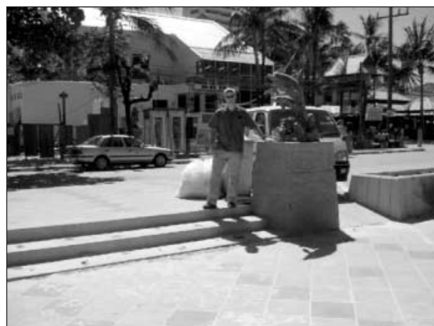
FIGURE 7 Pedestrian opening in the Patong Beach seawall (the short wall to the right of the figure). Tourist videos show that this wall deflected the tsunami run-up skyward, reducing forces on the seafront buildings.
