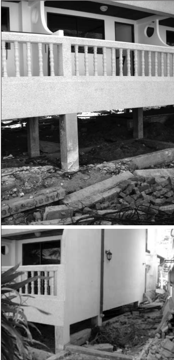
FIGURE 3 Two views of the Hotel Benjamin, Kamala Beach. The elevated structure escaped significant damage by allowing water to pass under it. The water level during the tsunami event was at the level of the exterior light fixture.
