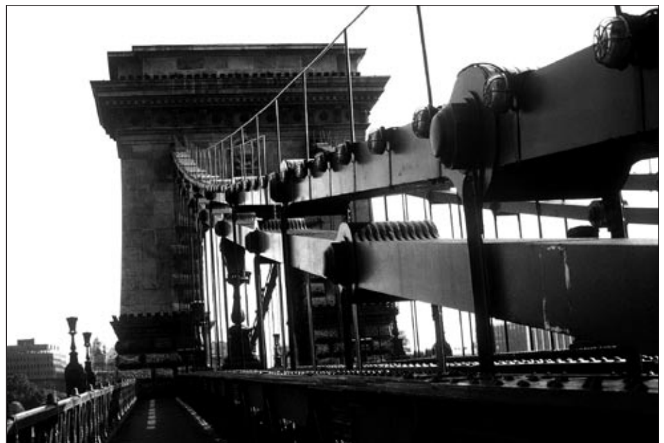
FIGURE 3 Eye-bars of the Budapest Chain Bridge.
