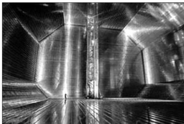
FIGURE 8 Main cargo tank of an LNG ship. Source: ConocoPhillips. Reprinted with permission.
