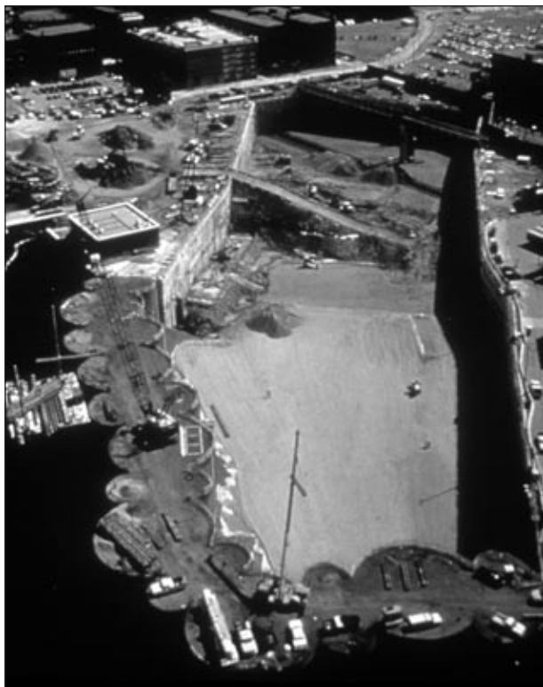
FIGURE 3 Casting basin constructed adjacent to Four Point Channel during Boston's Central Artery-Tunnel project, for manufacturing 30- to 50-ton concrete tunnel sections; when the sections were complete, the basin was flooded, and the sections were floated into position and submerged. The casting basin was 1,000 feet long, 300 feet wide, and 60 feet deep—big enough to hold an aircraft carrier or three Titanics side by side. (Photo: Massachusetts Turnpike Authority.)
