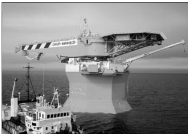
FIGURE 10 Fixed offshore ice-resistant offtake structure. Source: ConocoPhillips. Reprinted with permission.
