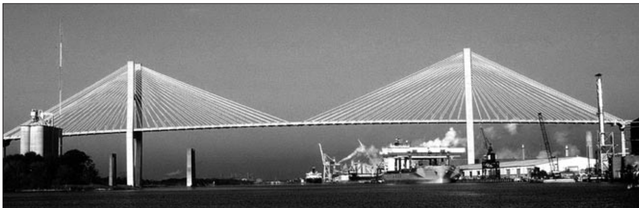
FIGURE 4 Cable-stayed bridge over the Savannah River.
