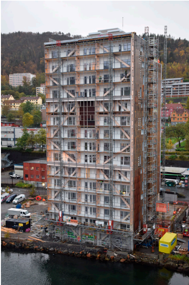
FIGURE 1 Treet, a 14-story apartment building in Bergen, Norway, rises 52.8 meters and is made of cross-laminated and glued laminated timber.
