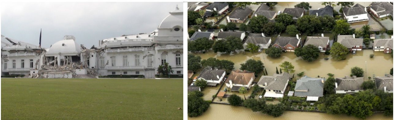
FIGURE 1 (left) The Haitian National Palace after the 2010 earthquake, which killed over 230,000 people and is considered one of the deadliest natural disasters in the Western Hemisphere. Photo by Reginald DesRoches. (right) Homes near Addicks Reservoir, west of Houston, after Hurricane Harvey, the costliest natural disaster in the United States in 2017. Photo by Philip Bedient used with permission.
